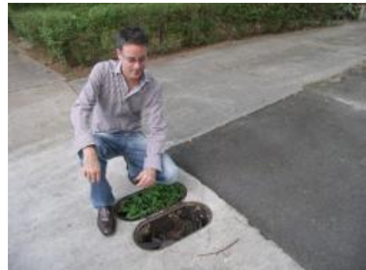
Midtown resident Mark Edge points out two water meter boxes with broken covers. Weeds grow in one.
