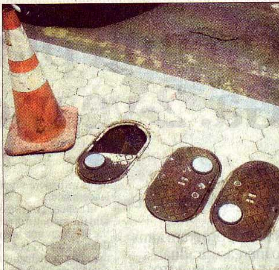
One of the water meter covers across the street from Taco Mac in Virginia-Highland is already broken, and the other two don't fit properly. John Becker For the AJC
